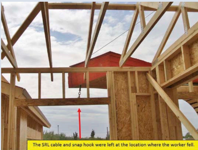
Photo 4: SRL cable and snap hook where fall was arrested. Note proximity to truss top chord and wall and path of lanyard over truss tail.
