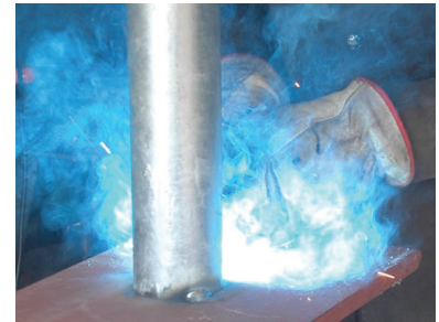
Field Welded to structural steel
