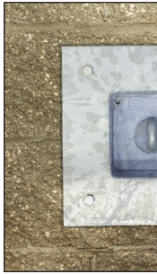
CMU Block Walls
