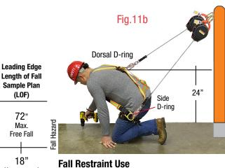
Fall restraint use shown at Fig.11b, requires guarding against falling over the leading edge. Use a warning line or other guarding method. The SRL connector "B" end may be attached to the dorsal D-ring or side D-ring of a full body harness.
