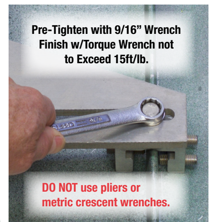
Fig.21 Base Plate Bolts
