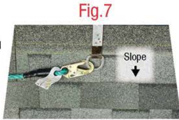
Side Loading Fall Restraint no Static Load
