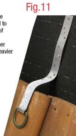
Conform Anchor Leg to the tile profile.
