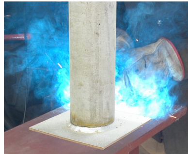
Fig. 11 Field Welded Base Plate
